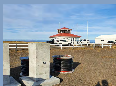
Installing PAPI lights in Blönduós Picture by Hjördis Þórhallsdóttir
